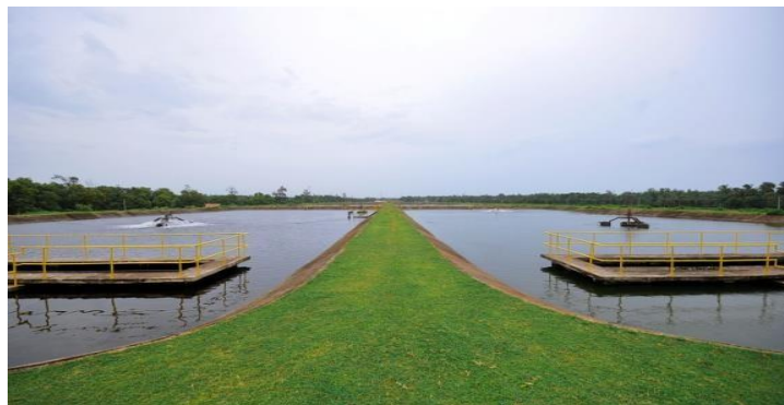
15 mld STP at Puri, Odisha
