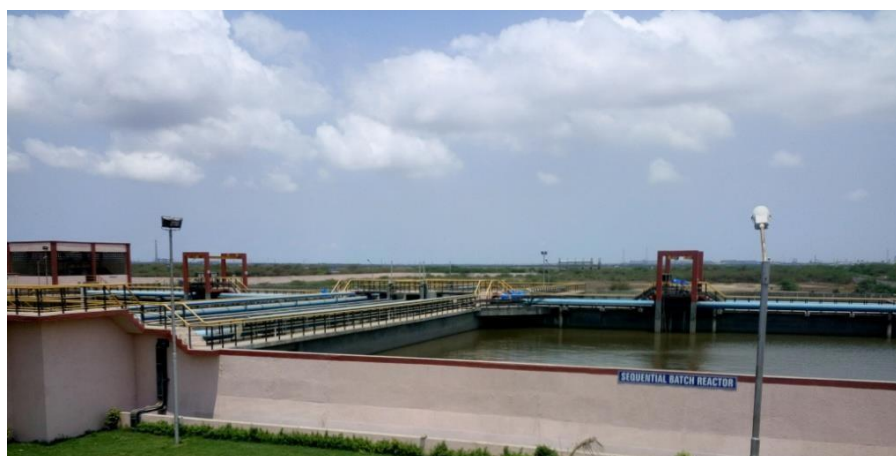
53 mld STP at Surat, Gujarat
