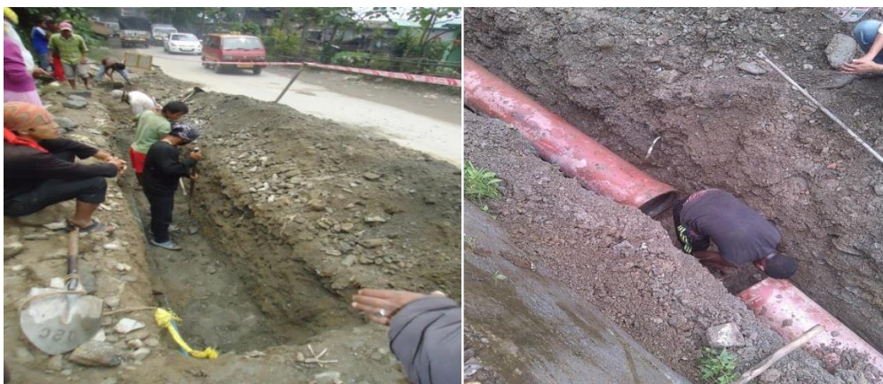
Sewer laying works under NRCP in Gangtok, Sikkim
